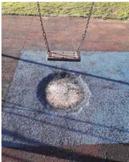
Soft landing areas under swings and chutes were pulled up with concrete exposed below.
