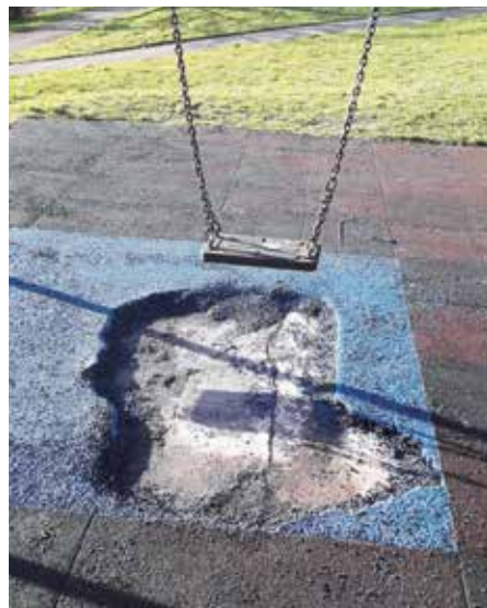
Soft landing areas under swings and chutes were pulled up with concrete exposed below.
